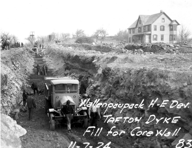
There's more to Wallenpaupack than meets the eye. This 1924 photo shows excavation for the impervious earth fill that has kept the Tafton Dike intact for more than six decades.
